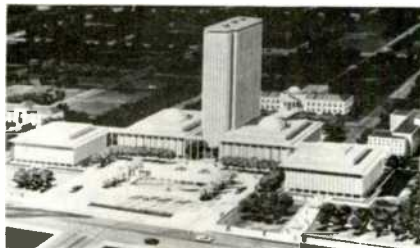
New capitol building under construction in Tallahassee.
