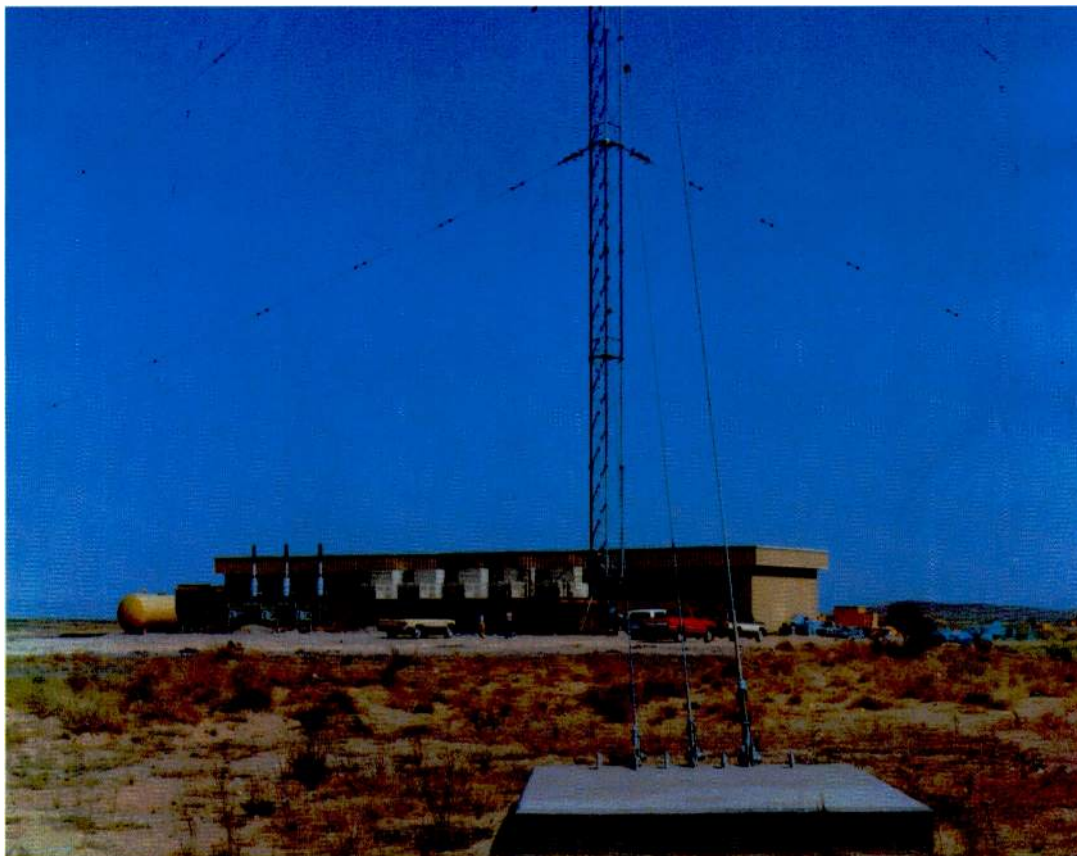
Transmitter station at Afif in Saudi Arabia.
