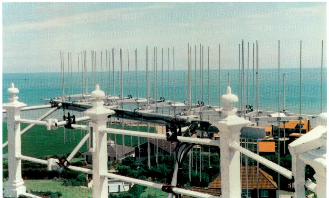
Radio lighthouse antenna mounted on the North Foreland lighthouse.
