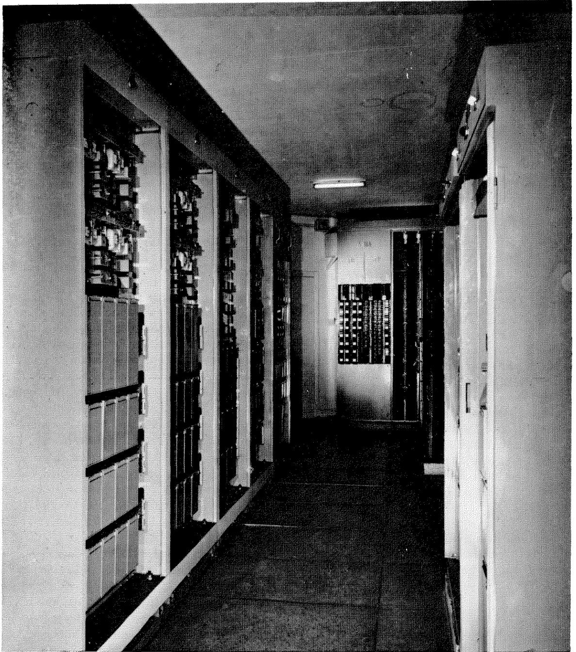
Figure 4—Racks of telecommunication switches at Algiers and terminations of cables to Arba.
