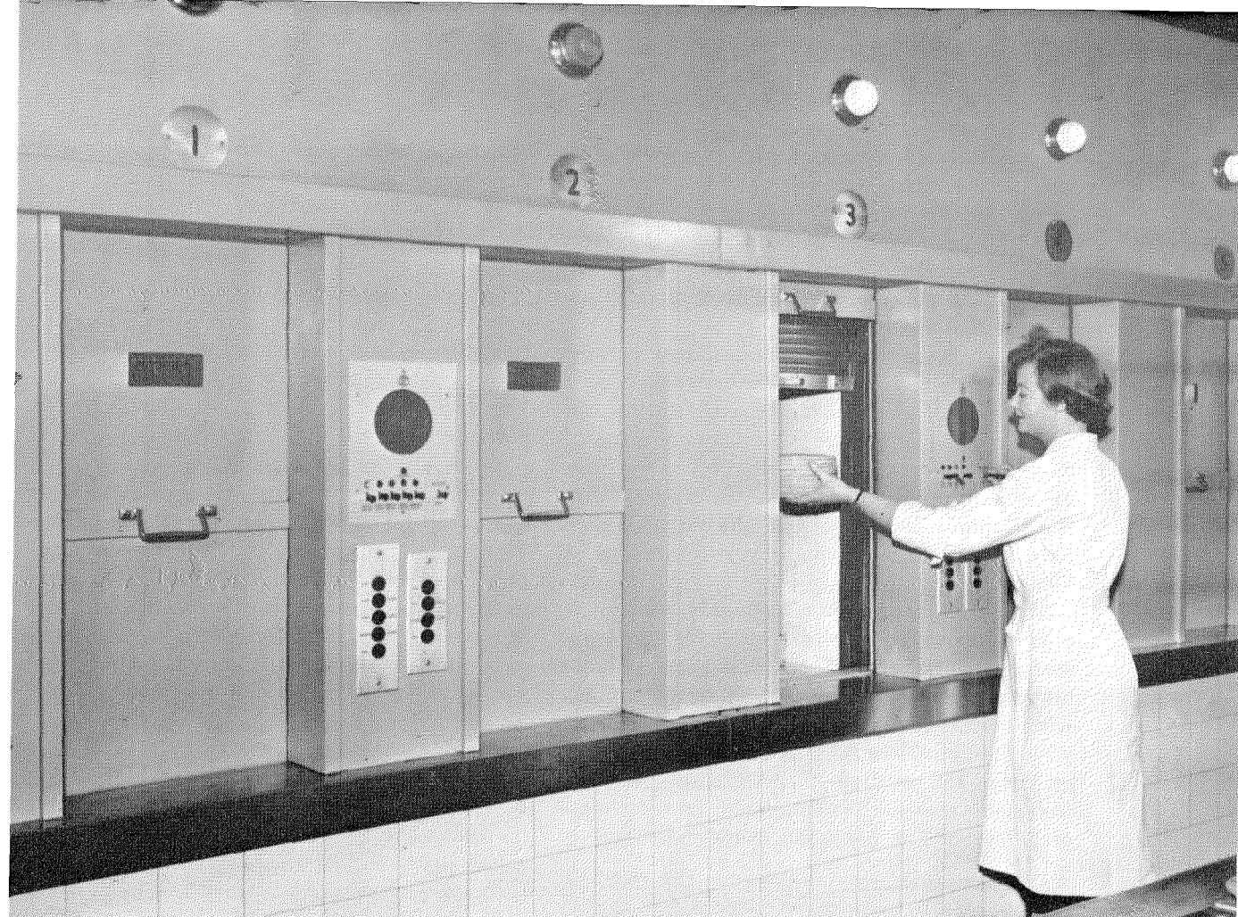
Completed installation showing lifts with intercommunication panels immediately above the lift-operation controls.
