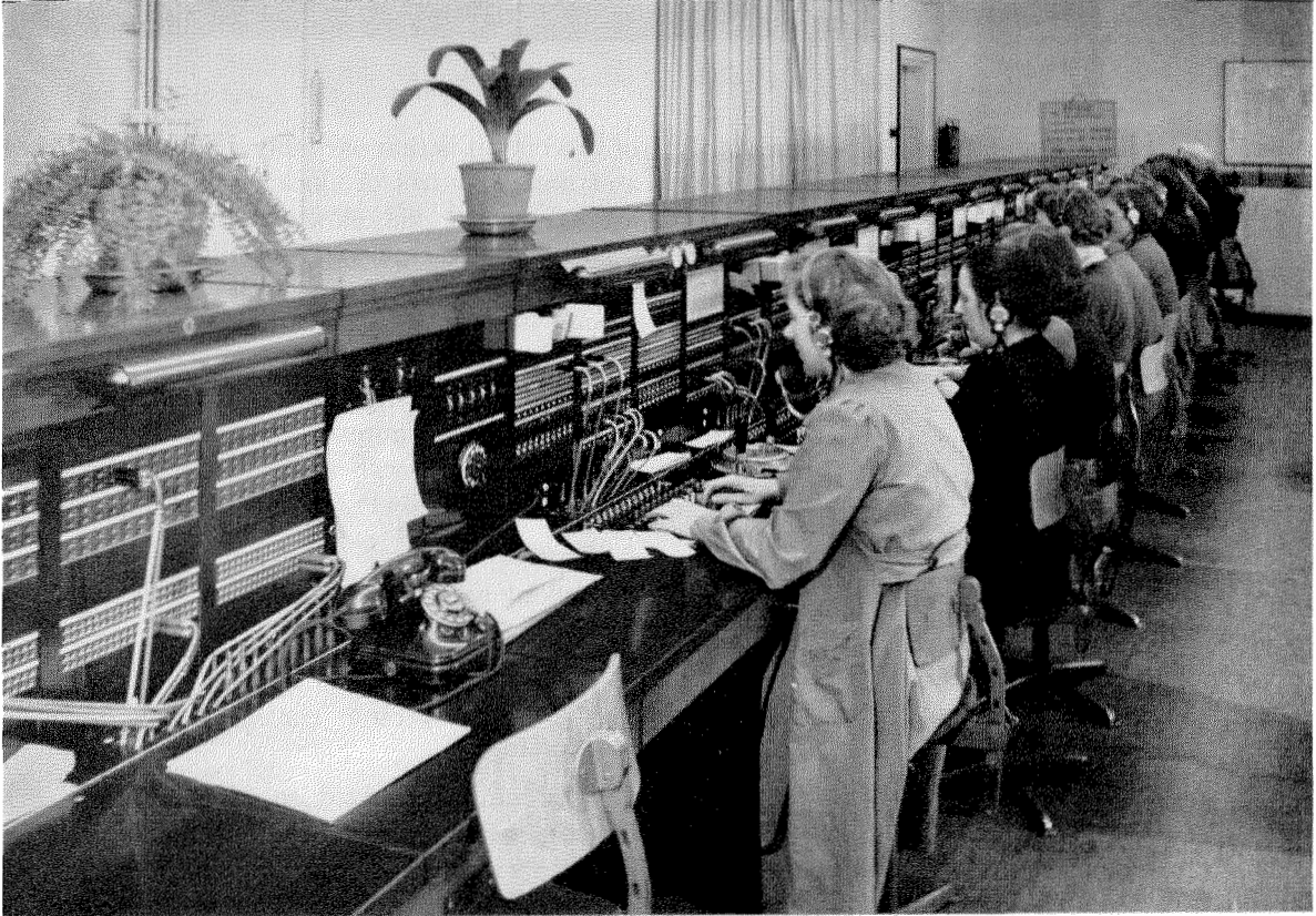
Figure 12—Toll operators in the Arnhem exchange.
