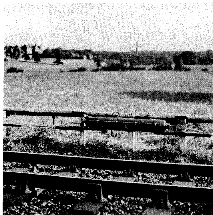
Figure 6—Pilot cables showing a loading-coil joint.
