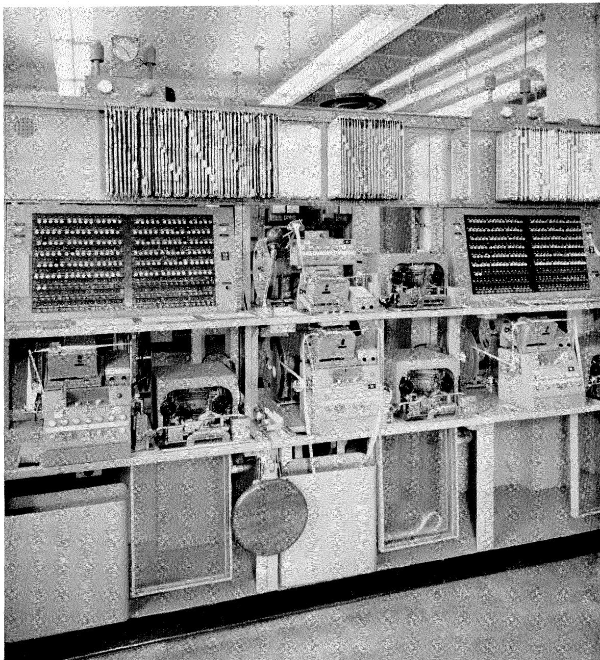
Figure 7—Push-button switching position.
