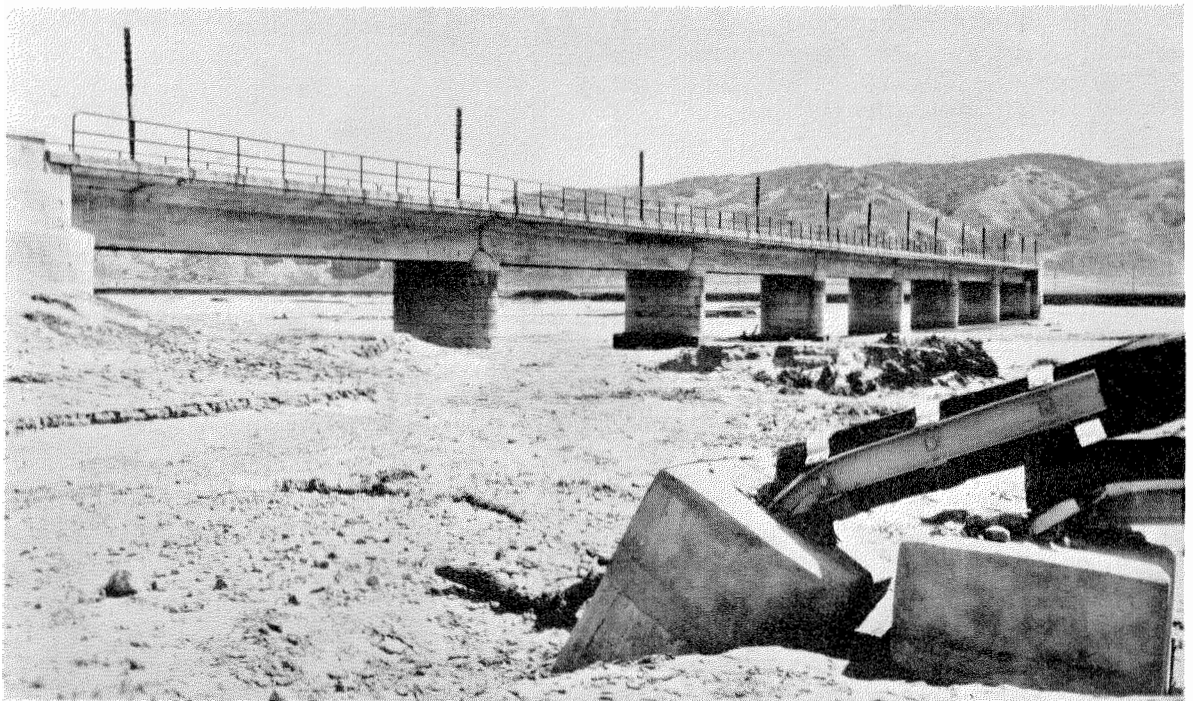
View of the bridge after the flood. Remains of one of the H structures are in the right foreground. All land between the end of the bridge and the distant right was washed out. The poles lashed to the bridge railing support the emergency lines.
