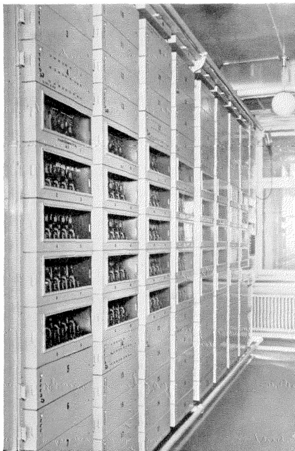
Fig. 5—Selective trunk circuits from 7-A1 local exchanges.
