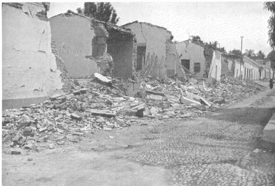
A Street in Colima After Partial Clearance.
