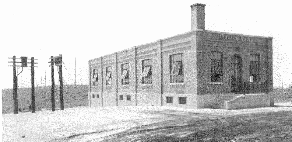
Fig. 4 A—Southampton Receiving Station, Point-to-Point Building.
