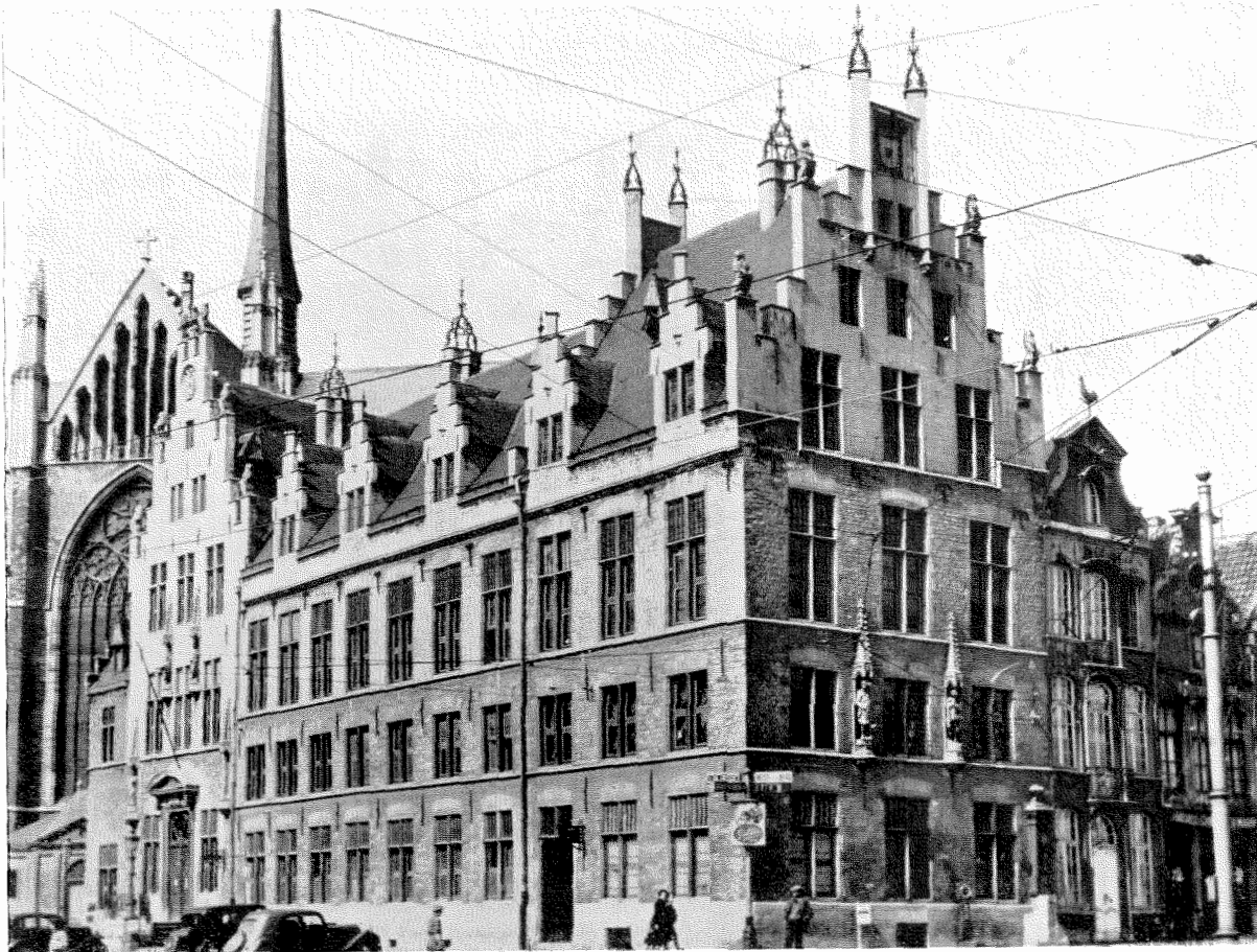
Situated close to Malines Cathedral, this building houses the new Malines Rotary telephone exchange, which is equipped for automatic ticketing. Subscribers of this exchange have full-automatic service to Brussels and Antwerp. All toll connections are recorded on tickets, which provide valuable traffic data and give a clear indication of the operating efficiency of the exchange.
