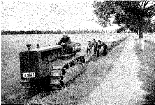
Trenching with Tractor-drawn Plough.
