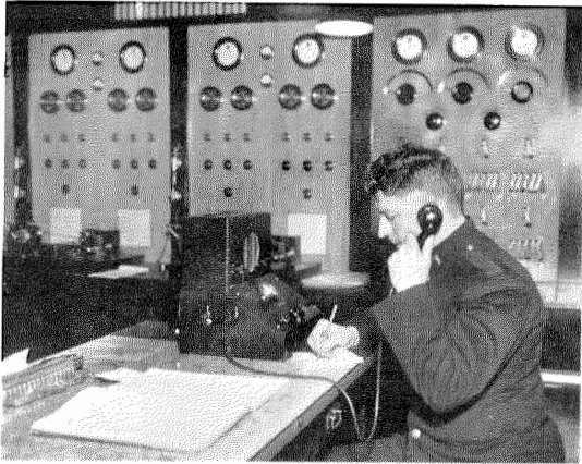
Fig. 4—Radio Telephone Switchboard Room at Headquarters.
