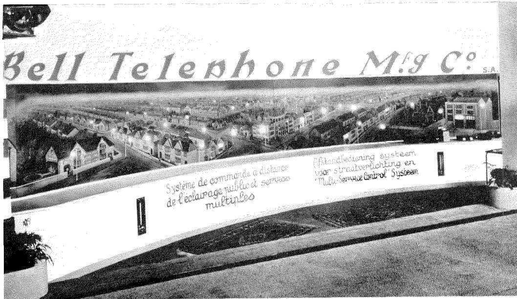
View of one side of the Bell Telephone Manufacturing Company's stand at the Brussels Fair, March 12th to March 26th, 1939, showing the exhibit of the remote control of street lighting and multi-service system.
