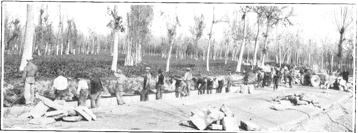
Figure 1—Cable-laying Near Naples.
