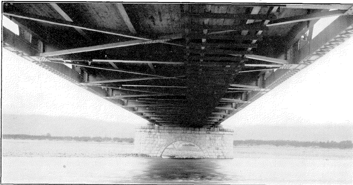
Figure 12—Toll Cable Placed Under Bridge—Oi River.
