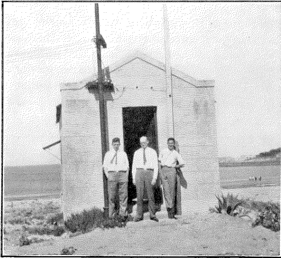
Cerro Cable Hut—Rawlings, Hubbard and King.
