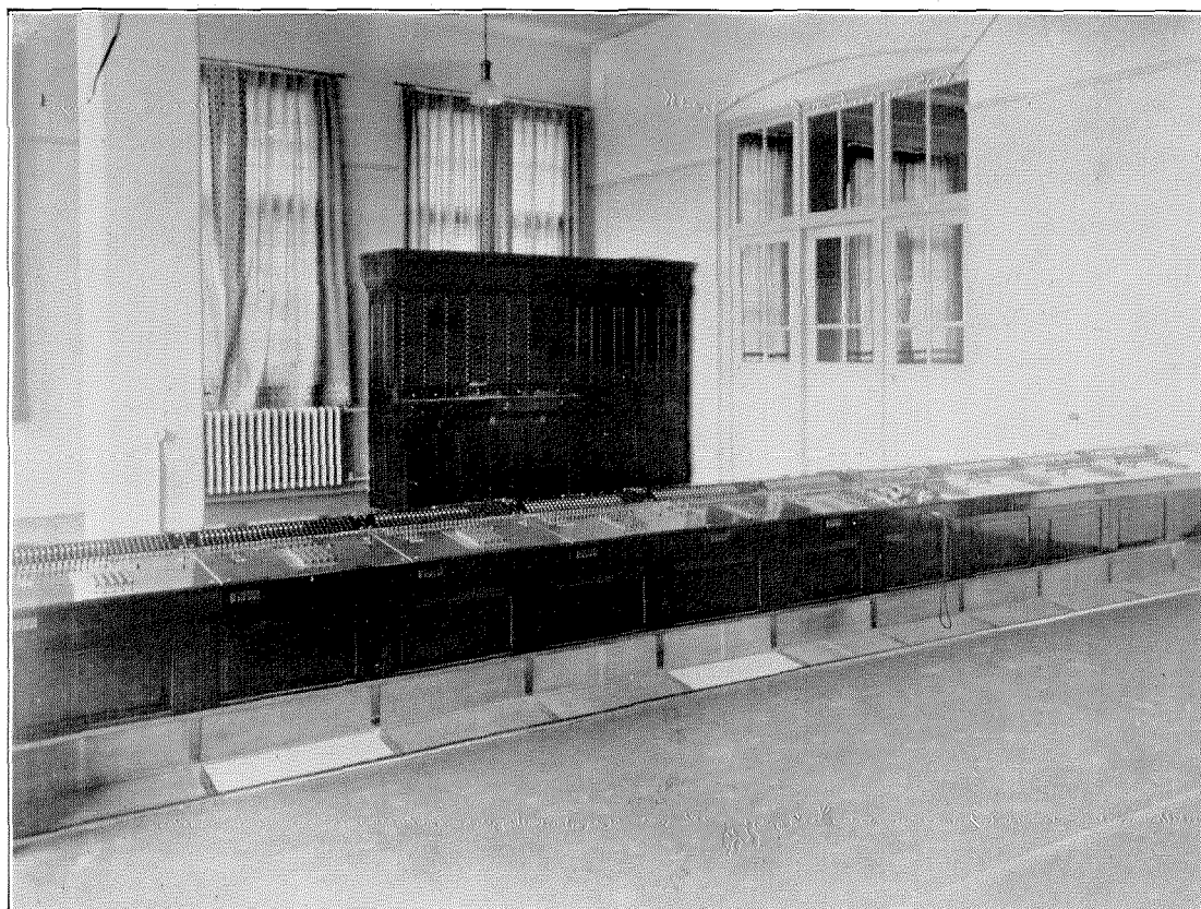
Figure 2—Scheveningen Exchange—Operators' Tables and Toll Switching Section
