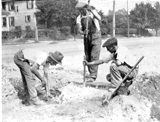
Figure 23—Manual Method of Breaking Concrete. Contrast with Figure 21
