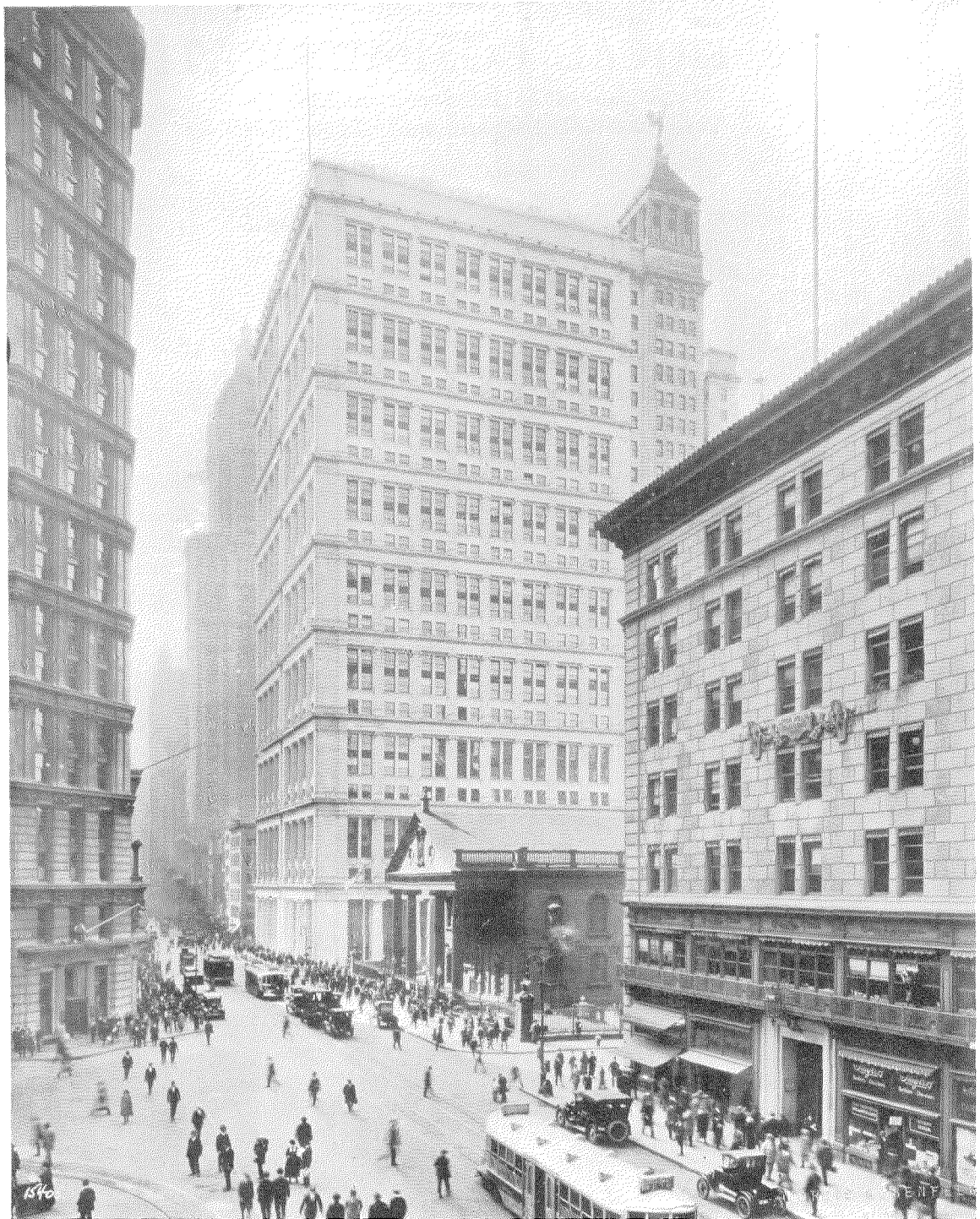
HEADQUARTERS American Telephone and Telegraph Company and Western Electric Company, Incorporated 195 Broadway, New York
