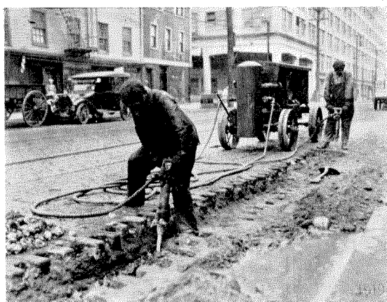
Figure 21—Removing Granite Blocks and Breaking Concrete Base
