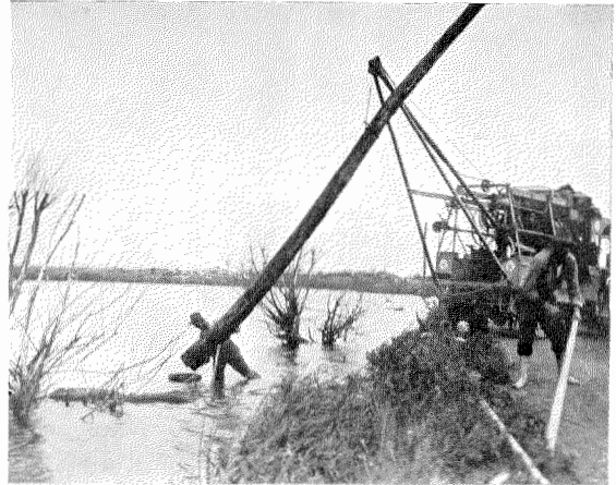
Figure 5—Derrick Operating Under Difficult Conditions
