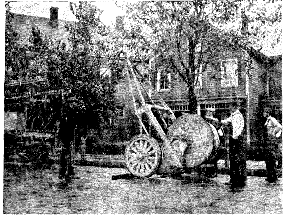
Figure 9—Truck Being Used to Load Reel of Cable on Trailers
