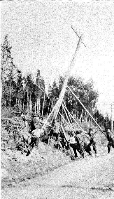
Figure 6—Erecting Pole by Manual Methods. Contrast with Previous Operations
