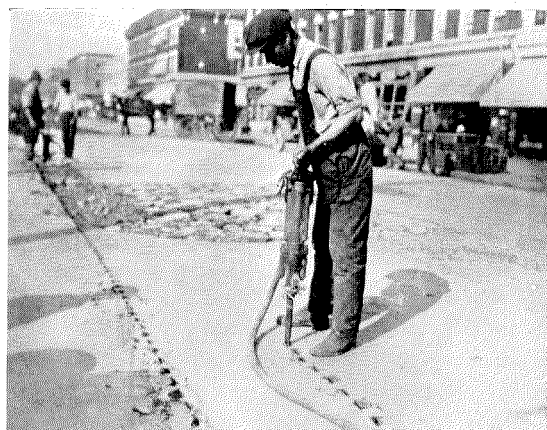
Figure 22—Air Gun Cutting Asphalt
