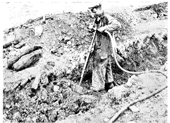
Figure 25—Pneumatic Spade Replacing Hand Pick Method of Loosening Hard Soil
