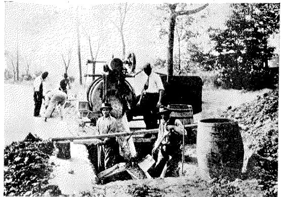
Figure 14—Pouring Concrete Manhole. Note 4-way Chute for Uniform Distribution
