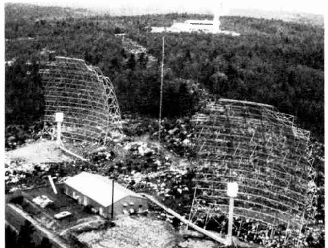
Fig. 8—A view of the Millstone Hill, Westford, Mass., terminal of the AN/FRC-47(XD-1) tropospheric scatter system.
