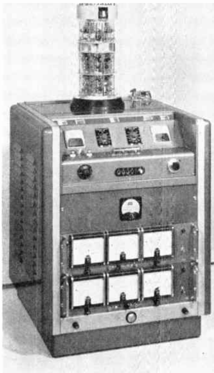
Fig. 28—Complete decoder terminal.
