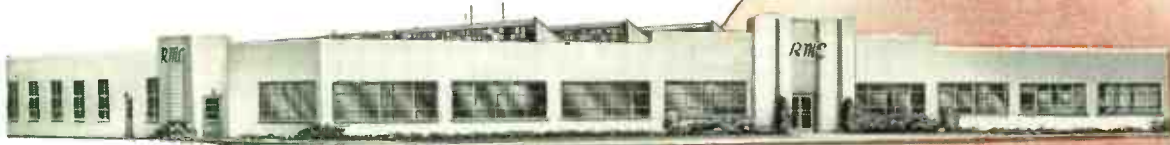
RMC Plant at Attica, Indiana
