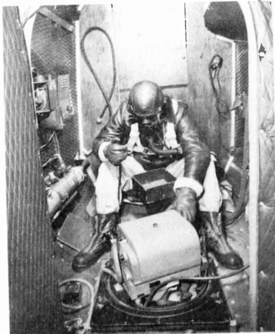
Fig. 1 Aerial photographer with camera and view finder installed in an airplane.
