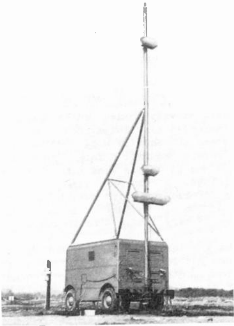
Fig. 11 - Glide-slope equipment.
