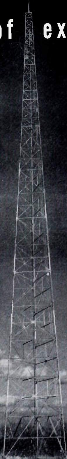
WPJB-FM-TV Broadcasting Station, Providence, R.I., using a Truscon Self-Supporting Radio Tower 431 feet high, to support an RCA-TV Double Antenna 2-Section Pylon 14.7 feet high.
