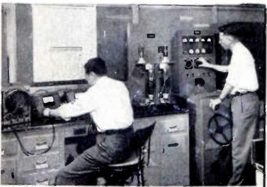
Testing modulation transformer under operating conditions
