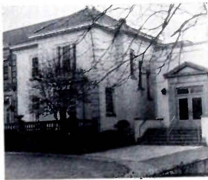
CINCINNATI ENGINEERING BUILDING
