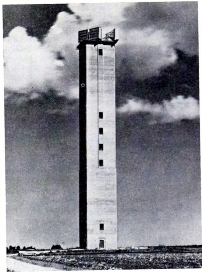
Fig. 15—A typical concrete station on the New York-San Francisco microwave radio-relay route. This station houses equipment developed at Bell Telephone Laboratories.
