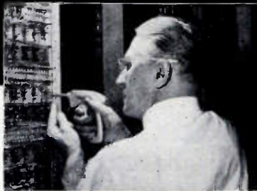
Bell Telephone Company craftsman wraps a wire to complete a connection. Wire is inserted into the nozzle and a rotating spindle whips it around terminals.
