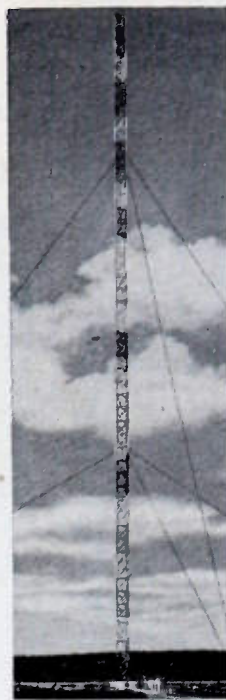
WHDH, Boston, Mass. Three Truscon Guyed Towers; 665 feet, 605 feet, and 645 feet high.
