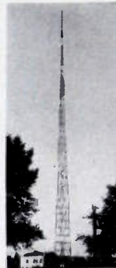
WTCH, Shawano, Wisconsin. Truscon Self-Supporting Tower, 240 feet high.
