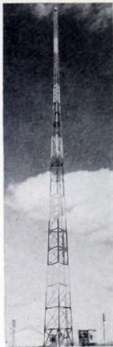
K A A-284, Owatonna, Minnesota, Northern Natural Gas Co. Truscon Self-Supporting Tower, 260 feet high.
