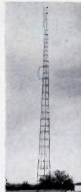
WMRI-FM, Marion, Indiana. Truscon Self-Supporting Tower, 336 feet high.
