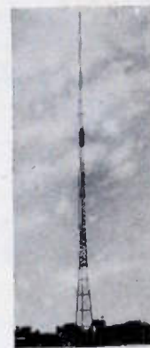
WEMP-FM, Milwaukee, Wisconsin. Truscon Self-Supporting Tower, 466 feet high.
