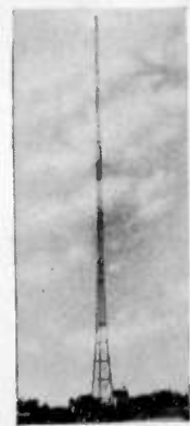
WEMP-FM, Milwaukee, Wisconsin. Truscon Self-Supporting Tower, 466 feet high.
