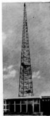
WXEL-TV Cleveland, Ohio. Truscon Self-Supporting Tower, 437 feet high.
