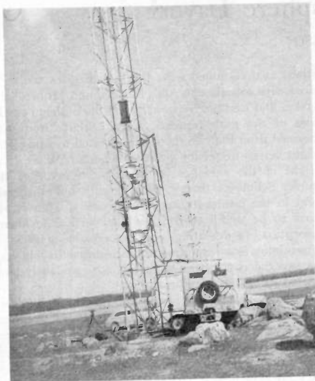
Fig. 9—The 60-foot tower and receiving truck.
