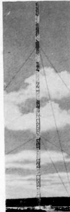
WHDH, Boston, Mass. Three Truscon Guyed Towers; 566 feet, 606 feet, and 645 feet high.
