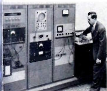
The three racks of laboratory equipment, plus recorders, and speakers, permit ensuring such performance characteristics as output at any frequency, uniformity of output at any frequency, signal-to-noise ratios, dynamic range, wow meter, harmonic distortion, intermodulation and modulation noise.
