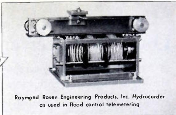
Raymond Rosen Engineering Products, Inc. Hydrecorder as used in flood control telemetering
