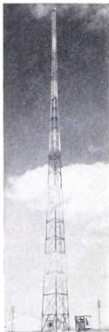
KAA-284, Owatonna, Minnesota, Northern Natural Gas Co. Truscon Self-Supporting Tower, 260 feet high.
