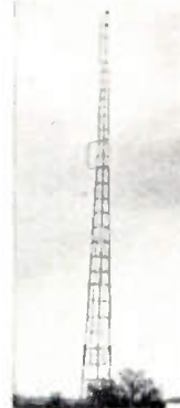
WMRI-FM, Marion, Indiana. Truscon Self-Supporting Tower, 336 feet high.
