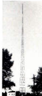
WTCH, Shawano, Wisconsin. Truscon Self-Supporting Tower, 230 feet high.
