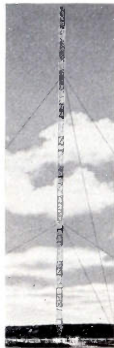
WHDH, Boston, Mass. Three Truscon Guyed Towers; 565 feet, 605 feet, and 645 feet high.
