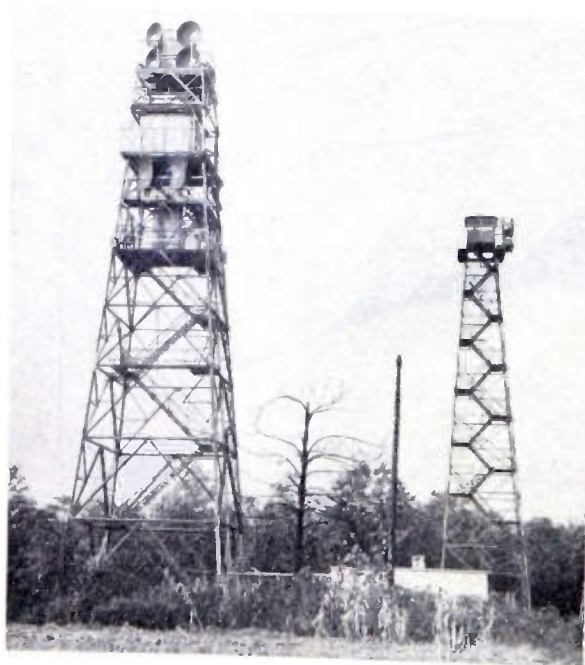
Fig. 3—Neshanic main radio beam tower (left), and propagation tower (right).
