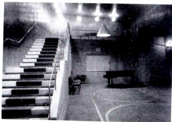
Fig. 8—Small-sized studio for speech and drama in the Norwegian Broadcasting House. The stair has three types (acoustically) of tread and the removable panels expose a gravel walk, a wood surface for tap dancing, and a marble surface for producing the sound of footsteps.
