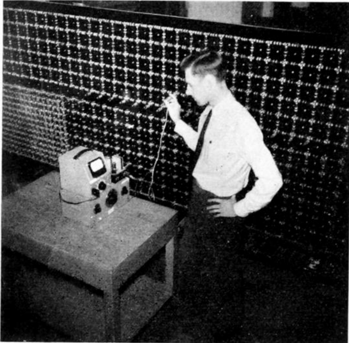
Fig. 4—Cylindrical-co-ordinate network in operation.
