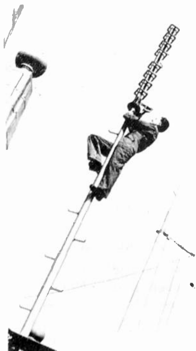
Fig. 3—Omnidirectional eight-loop transmitting antenna for the experimental multiplex broadcasting system, located at 67 Broad St., New York, N. Y.
