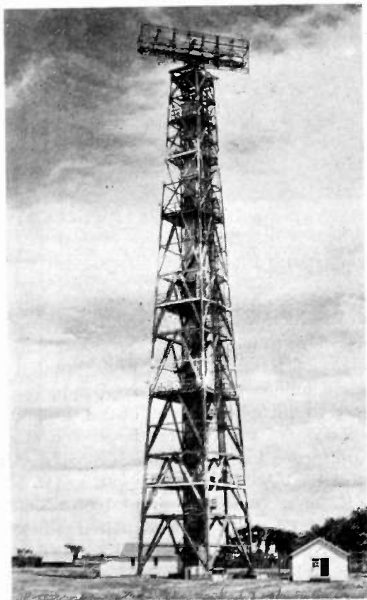
Fig. 9—Long-range early-warning station. The height-finding or VEB array can be seen on the side of the tower.
