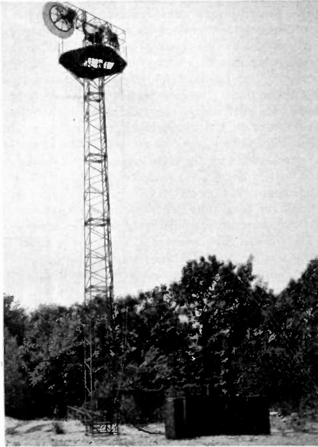
Fig. 3—Radio Set AN/TRC-6 including stand-by (spare multiplex and radio) units. Note that the radio-frequency units are mounted on the antenna reflectors.
