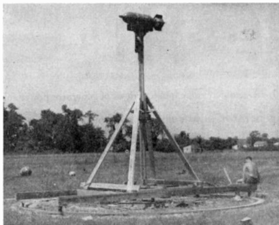
Fig. 6—Structure used for obtaining directivity envelope for proximity fuze.
