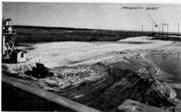
Fig. 13—Proximity-fuze proving ground, with rocket firing tower at left and a simulated bomber at right.
