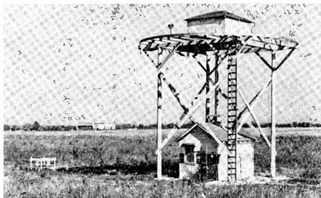
Fig. 16—Two-course radio range with sector identification and simultaneous voice, showing transmitter house, counterpoise structure, antenna house, and 125.020-megacycle marker.
