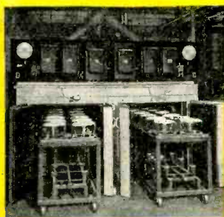
Baking screens and wall coating
