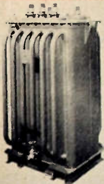
150 KVA Distribution transformer, single phase, 600 high voltage, 240/120 low voltage.
