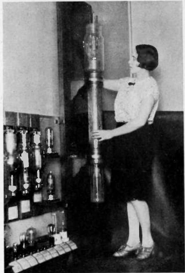
Fig. 6—100- to 200-kilowatt Westinghouse AW-220 tube.
