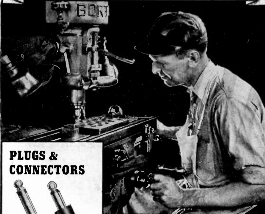
Remler craftsman die-sinking a multiple mold for Signal Corps Connectors
