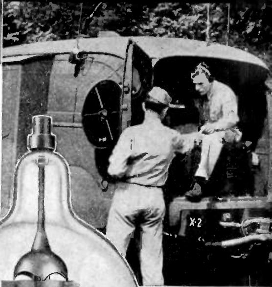
Complete High Power Radio Transmitter and receivers mounted in light army truck. These transmitters are in service in all theatres of war and in most all branches of the army.
