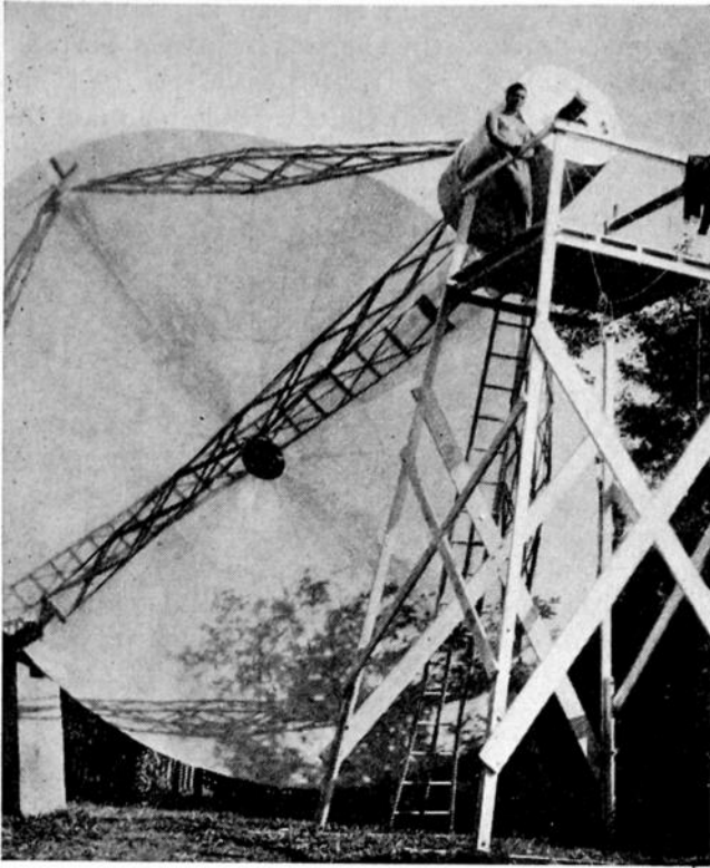
Fig. 2—Collector pointed to declination -32.5 degrees. Large drum at focal point for operation at 160 megacycles.
