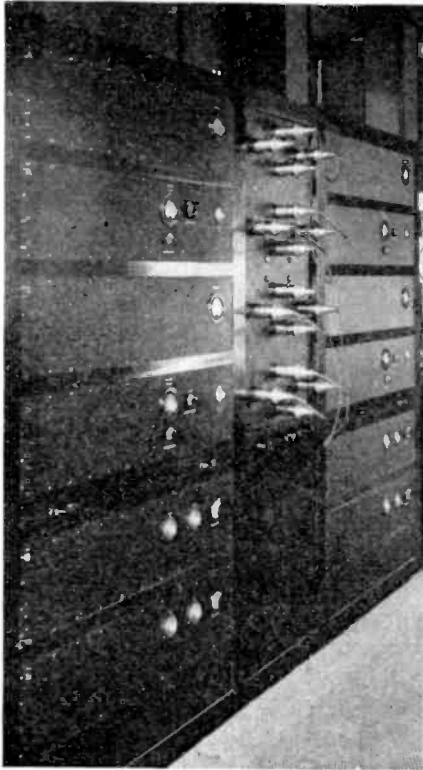
Fig. 7—Radio-Koorwijk. Second modulation stages and distributing panel to transmitters.
