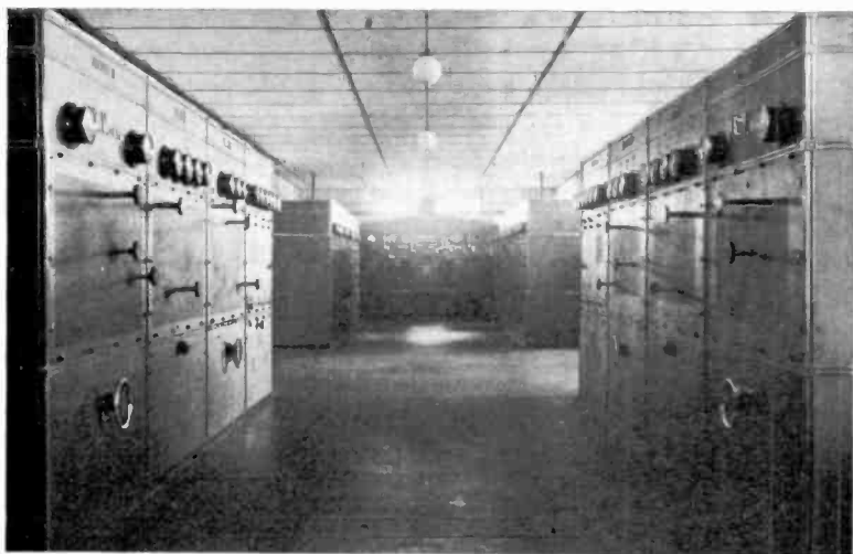
Fig. 5—Radio-Kootwijk. General view of the four single-side-band transmitters.
