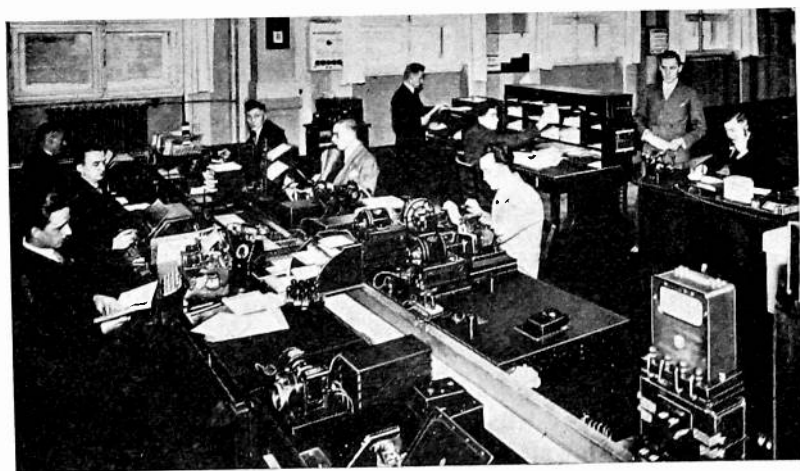
Fig. 9—Operating room of the operating central office, Hamburg.
