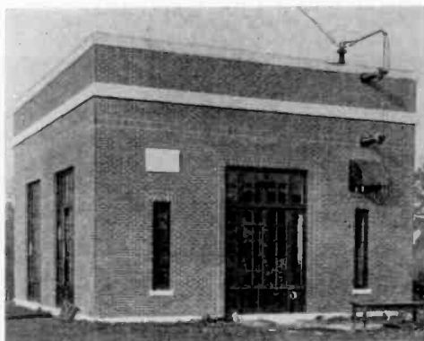
Tube transmitter house. NSS. Showing lead-in for transmitting and ice melting.
