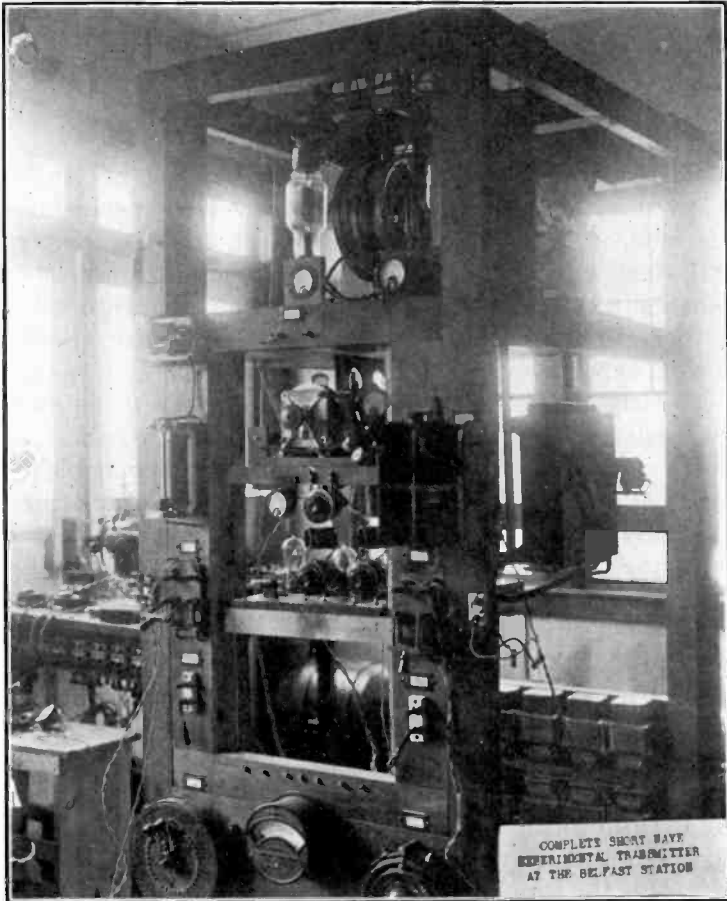
Figure 1—Experimental short wave radio relay transmitter 2XAO—Belfast, Maine.
