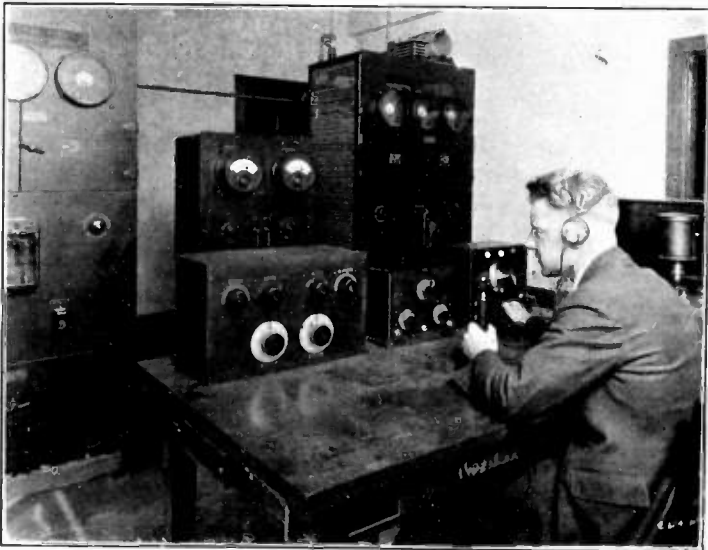
FIGURE 45—Washington Broadcasting Station Operating Room, Showing Control Desk, Duplicate Transmitters, and Filter Panel
