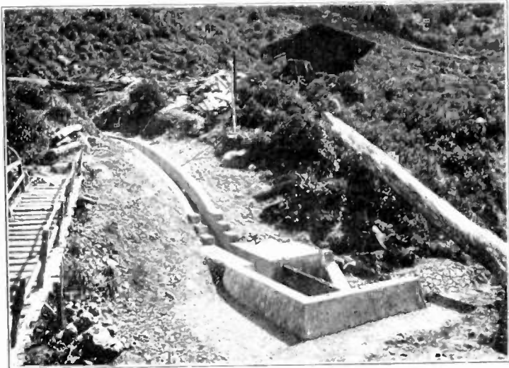
FIGURE 7—End of Tunnel with Open Conduit to First Reservoir
