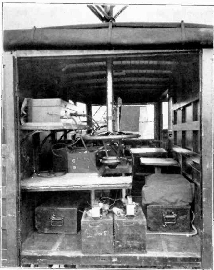
FIGURE 19—Interior View of Truck Installation
