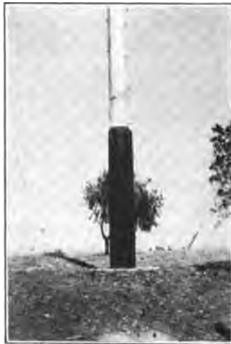
FIGURE 20—View of the Special Footing for the Masts
