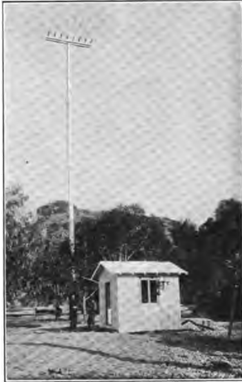
FIGURE 21—View of the Transmitter House, Showing the Mast and Antenna Construction
