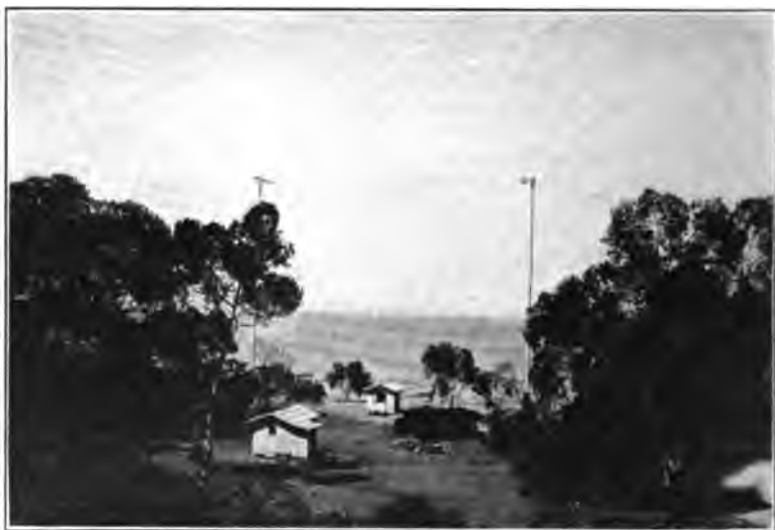
FIGURE 22—View of the Antenna System at Pebbly Beach
