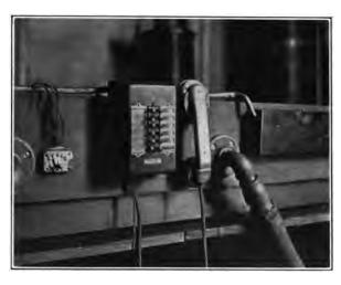
FIGURE 22—Telephone Intercommunicating Station for Wire or Radio Communication
