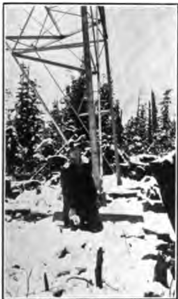
FIGURE 3—"Tower C," Ketchikan Radio Station
