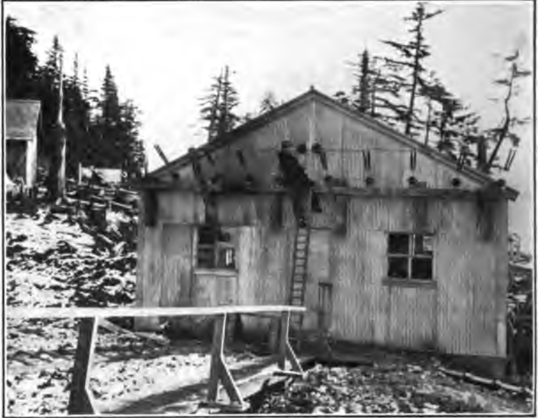
FIGURE 2—20 wire aerial terminal, showing high tension porcelain insulation, 20' wood strain insulation, and 2 Bradfields
