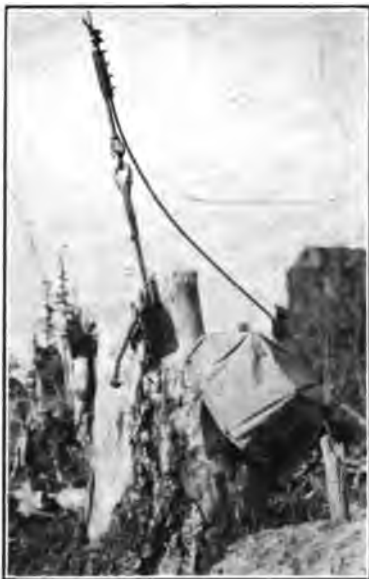
FIGURE 4—Tower safety stops, showing complete arrangement, (winch or crab, and the galvanized iron nailed to top of stump to preserve the same. Note steel halyard slack; Manila links shackled to a short piece of steel halyard which in turn is clamped to the halyard; ship cleat bolted to stump with 12" lags. Ketchikan.
