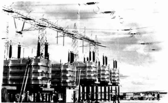
[4] Converter valves erected on site with buswork.
