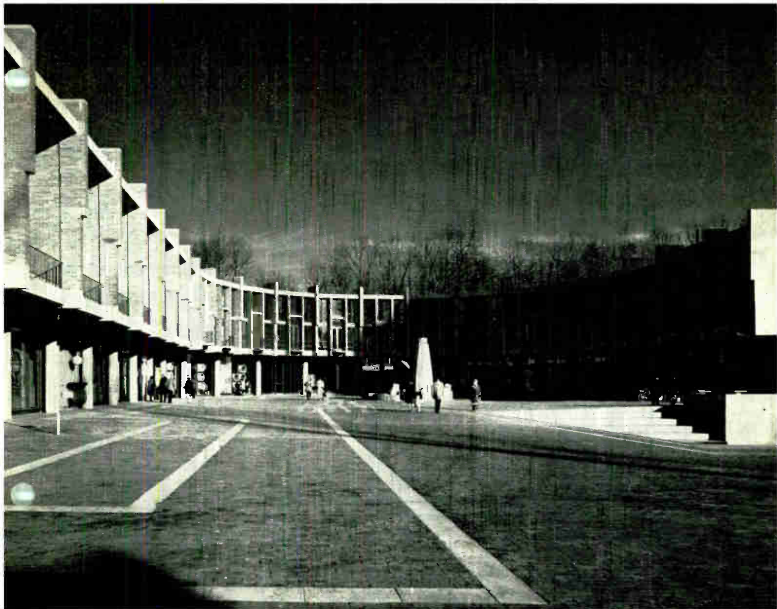
FIGURE 3. View of Reston's horseshoe-shaped shopping plaza. Specialty shops occupy street-level space. Professional offices and apartments are located on the second and third floors of the structure.
