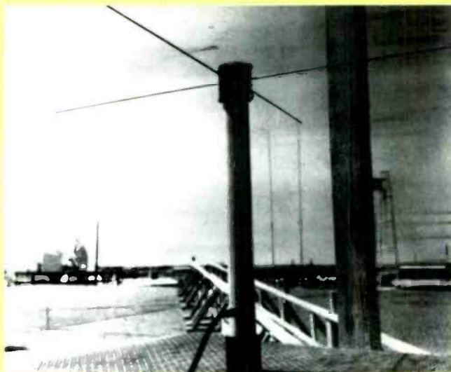
The satellite receiving antenna shown here is identical to one used by the author. The roof site is a commercial plant that requires satellite reception for accurate weather information. Even the pros use the author's home-brew antenna.
