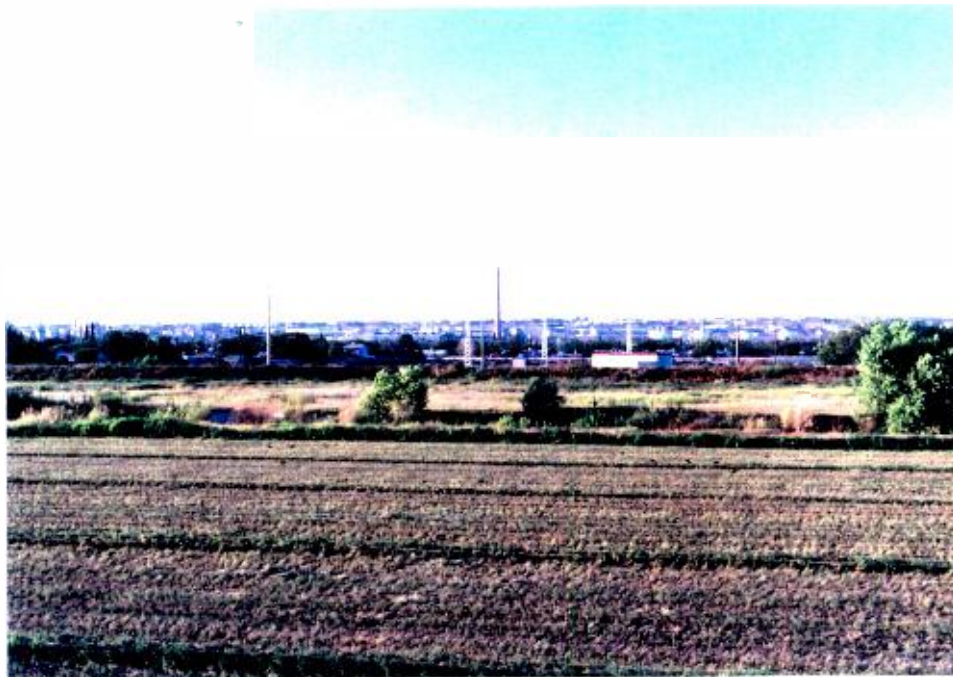
View of KELP site taken from Mexico. Rio Grande River appears as "ditch" in foreground; street lights and security camera are along the Chamizal Border Highway on the U.S. side. The KELP towers are visible as well as a chimney and other structures.
